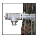
9. TEFLON tape the threads of the nipple installed in the outgoing tee then thread the outgoing tee into the side of the Steam-Away. Tighten with the clampable end vertically down. Note: Depending on the installation it may be necessary to remove the 2" plug from the coupler. If this is done, ensure there is a plug in the coupler located on the other side of the Steam-Away.
