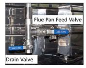
1. Close the Steam-Away drain valve and open the feed valve for the flue pan.
