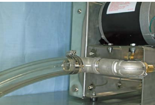
Completed Input Hose Connection
