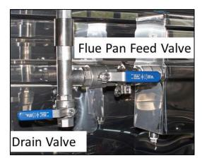
1. Close the Steam-Away drain valve and open the feed valve for the flue pan.
