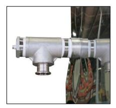
8. TEFLON tape the threads of the nipple installed in the outgoing tee then thread the outgoing tee into the side of the Steam-Away.
