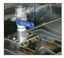
8. Thread a 1" stainless steel ball valve (not included) onto the stainless steel nipple. Tighten the ball valve into a position where it can work freely.
